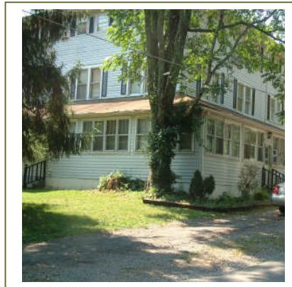
Eight Unit Apartment Building on the Corner of Magnolia and Sterling Street in Maryville, Tennessee
